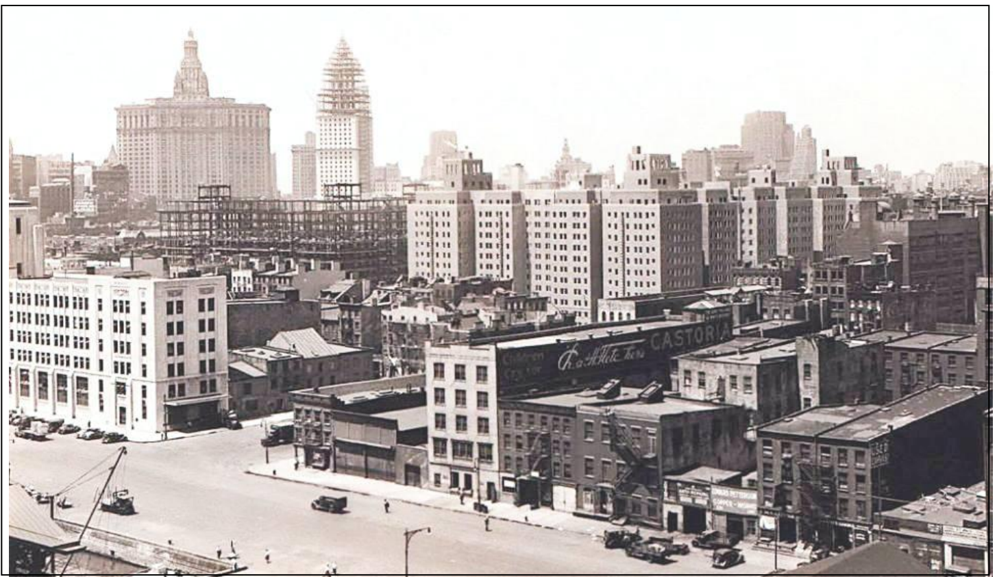
The construction of Knickerbocker Village, as seen from the Manhattan Bridge, 1933.
