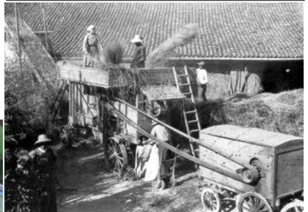
Arduous Task —The mechanical thresher that was introduced in the 1950's was a magnificent improvement over the arduous task of flailing the
